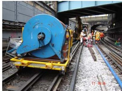
**Figure 12 – hydraulically-powered cutter unit on rail flatcar**
