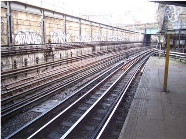
**Figure 2 – View eastwards from platform of disused Kings Cross station (note catch pit between roads in lower left foreground)**
