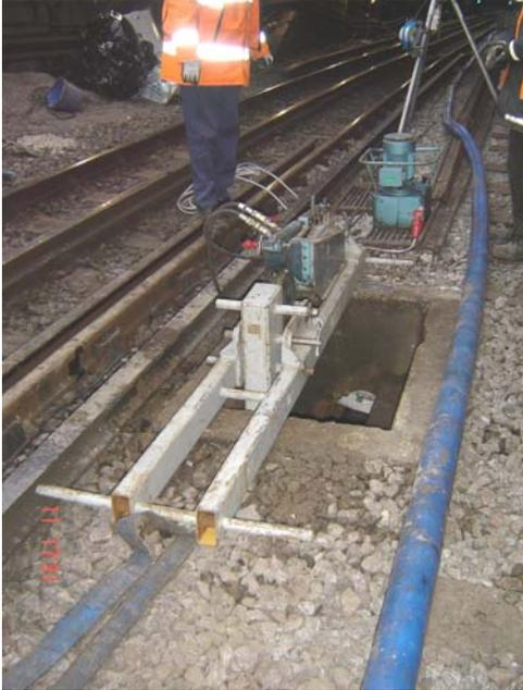
**Figure 9 – Tirfor winch and boom arrangement**
