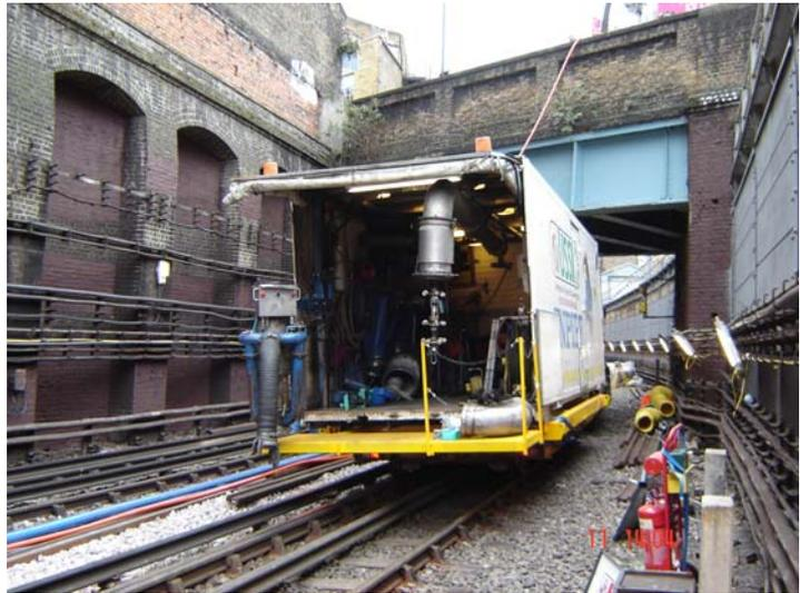
**Figure 10 – Inpipe unit positioned for liner curing**
