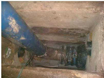
**Figure 11 – Inpipe liner inflated and curing in progress**
