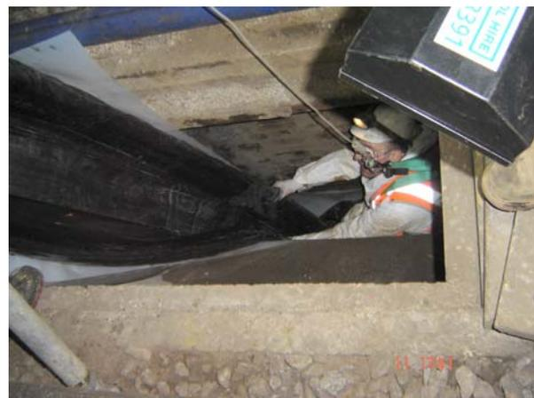
**Figure 8 – Inpipe liner insertion**
