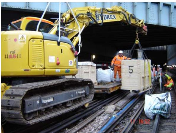
**Figure 7 – unloading Inpipe product crate at point of use**
