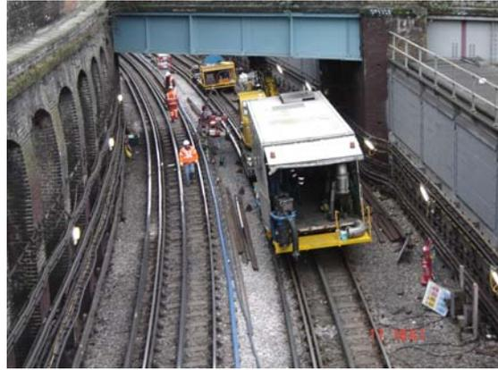
**Figure 6 – Inpipe equipment container loaded onto roadrailer flatcar**
