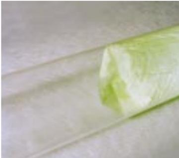
We insert the liner on site using compressed air
